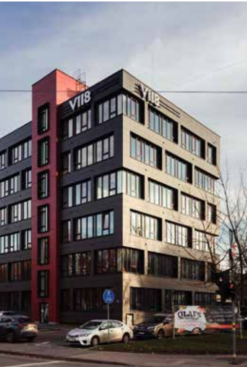
COMMISSIONING OF THE OFFICE BUILDING “V118” RIGA, LATVIA
