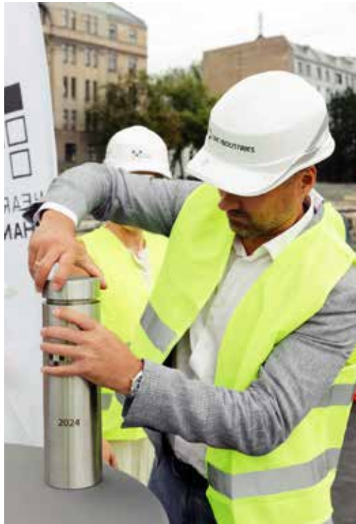
SEALING OF THE TIME CAPSULE IN THE FOUNDATION OF “HEART OF HANZA” RIGA, LATVIA
