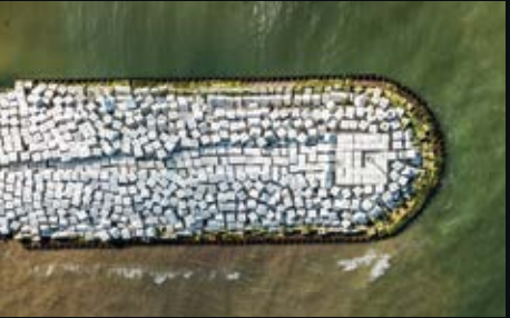
CONSTRUCTION OF A GROYPE SEASHORE PROTECTION STRUCTURE NEAR LIEPAJA IN LATVIA.
