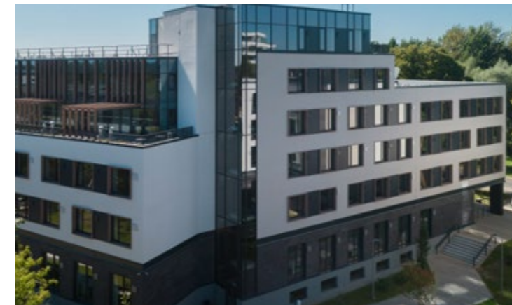
Construction of the modern student hotel at 8 and 12 Jelgavas Street in Riga, Latvia
