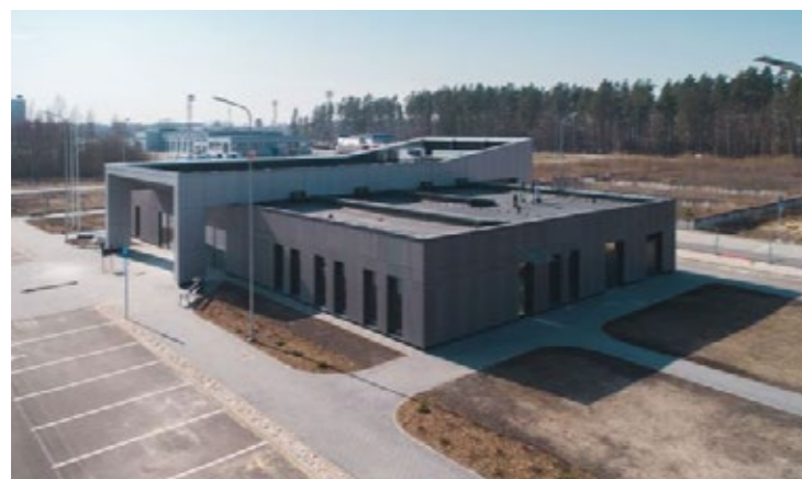
Construction of the Road Traffic Safety Directorate's Customer Service Centre Jelgava, Latvia
