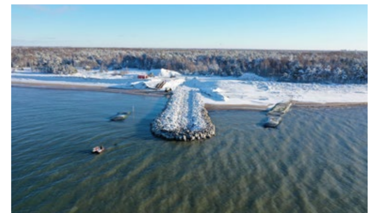
Jetty marine structure to reduce coastal erosion in Liepāja, Latvia
