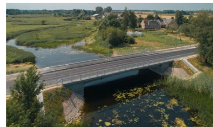
Reconstruction of the Svētes Bridge on Road P95 at the Jelgava-Tērvete-Lithuanian border (Žagare) in Jelgava municipality, Latvia
