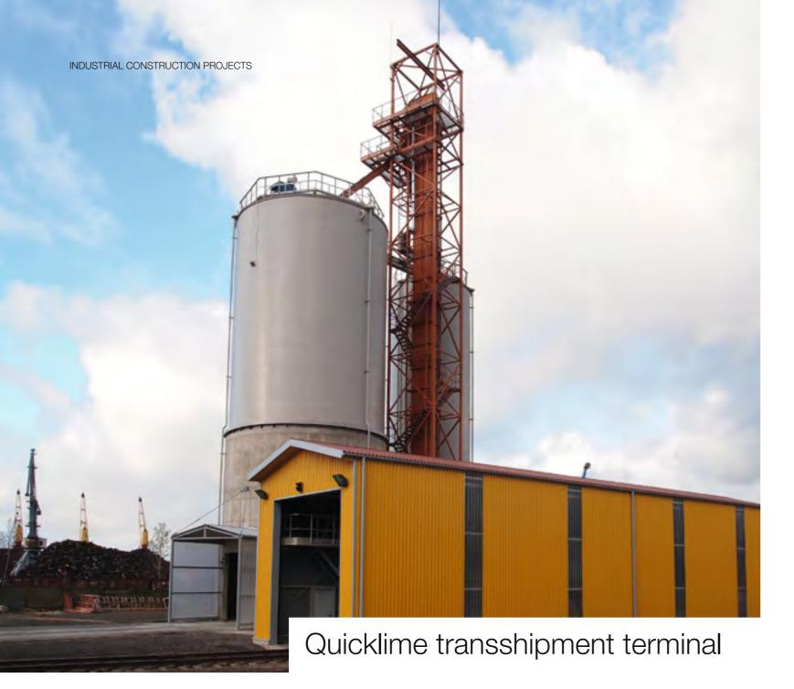
The quicklime transshipment terminal in Liepaja was designed, built and commissioned on a turnkey basis by LNK Industries. The terminal comprises not only facilities, but also a transshipment system for quicklime delivery and handling, as well as an automated control system.
